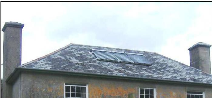
The solar tubes contribute to the domestic hot water requirement and also to space heating for both the cottage and the house via the downstairs underfloor heating. The installations include temperature monitoring and Nu-heat hot water tanks with solar coils.
