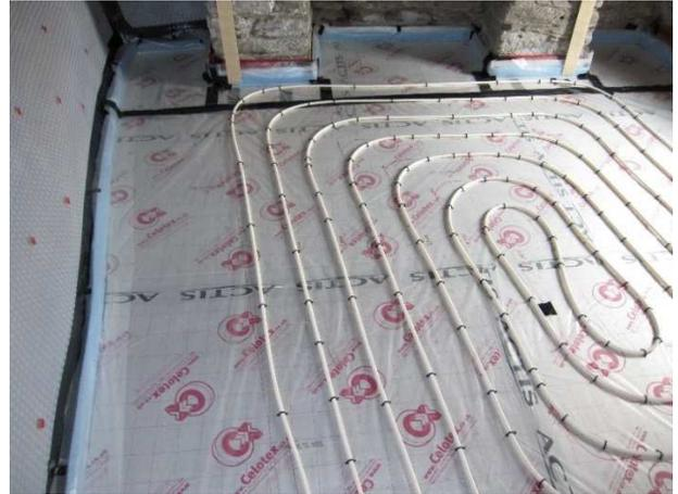
45 mm thick Isocrete self-levelling screed (installed by J H Lidstone Ltd of Plymouth) covers the pipes and spreads heat in the floor plate
