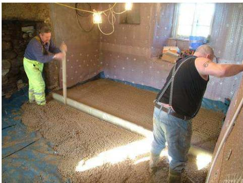
Therefore the inside face of the walls were 'sealed' in affected areas using two very different types of tanking:
