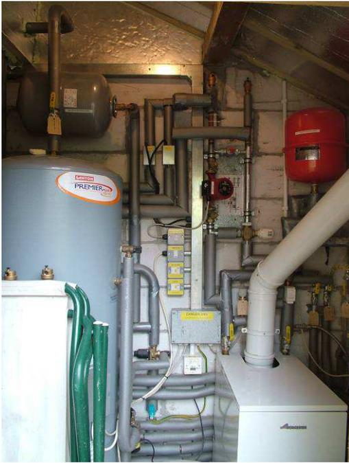
modern oil condensing boiler with an efficiency of about 93% (reducing fuel use per kW by 20 to 30%).
